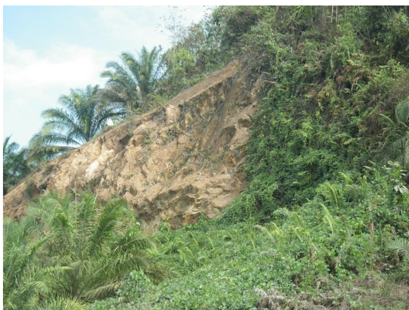
Landslide in an oil palm plantation
