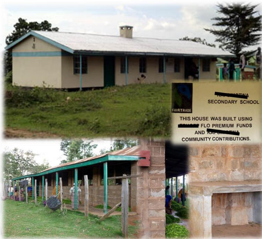
Examples of FT Premium funded investments: Teachers' housing to attract good teachers; fencing, electricity and water installation at collection centre; concrete sorting benches.
